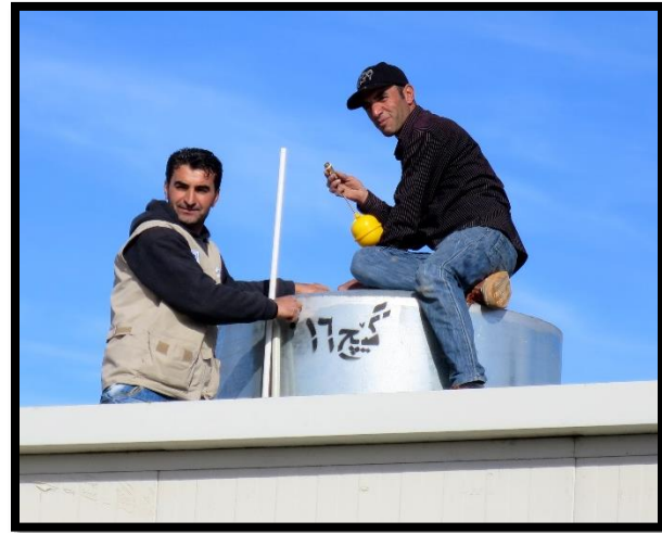
Minor Fixers Working on Health Center Tank
