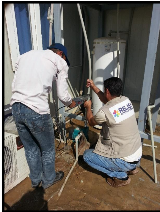
Minor Fixers addressing HH supply issue
