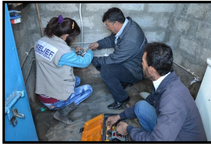
Minor Fixers Changing the Faucet (Mixer) in a HH
