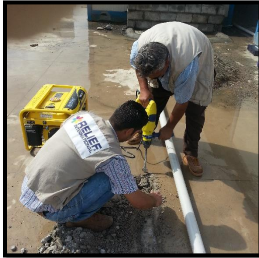
Minor Fixers repairing school water supply pipe
