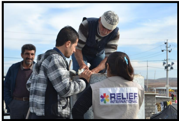
Minor Fixers working on a HH water tank
