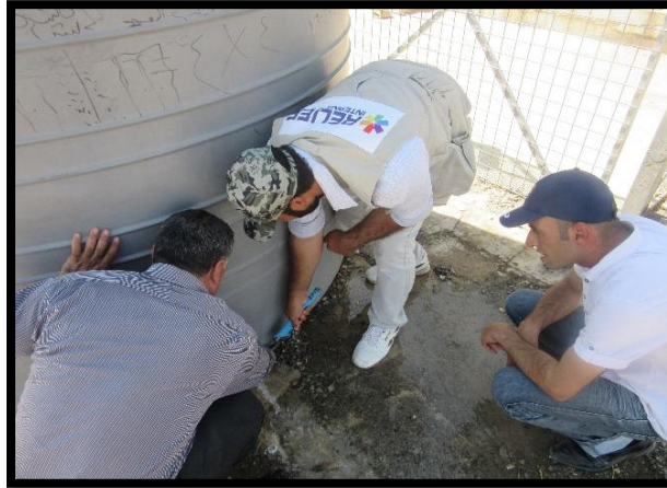
Minor Fixers repairing health center water storage tank
